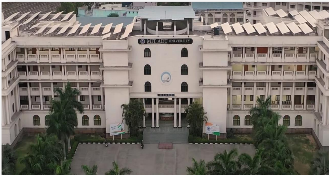
Solar panels on roof top of MANET Building
