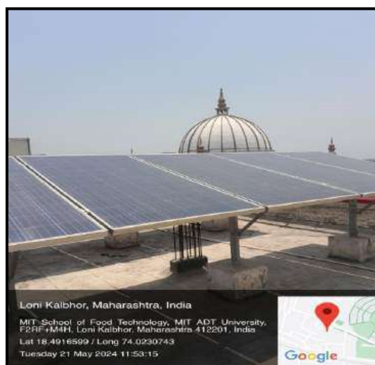
Photograph of Solar PV Plant & Solar Thermal Water Heating System:
